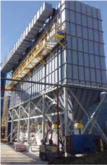
C.P.E. Filters' 5-Module Baghouse
